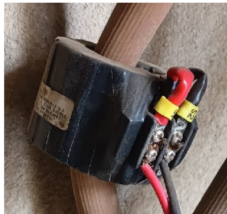
Fig 3.5 current transformer
