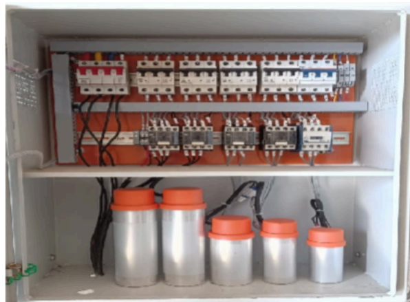
2. Interior view of panel
